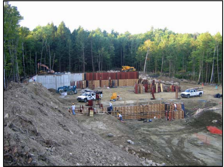
DRTC construction site as of September 9, 2005
